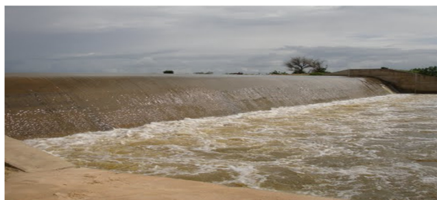
Fig. 1. Alau Dam Maiduguri
